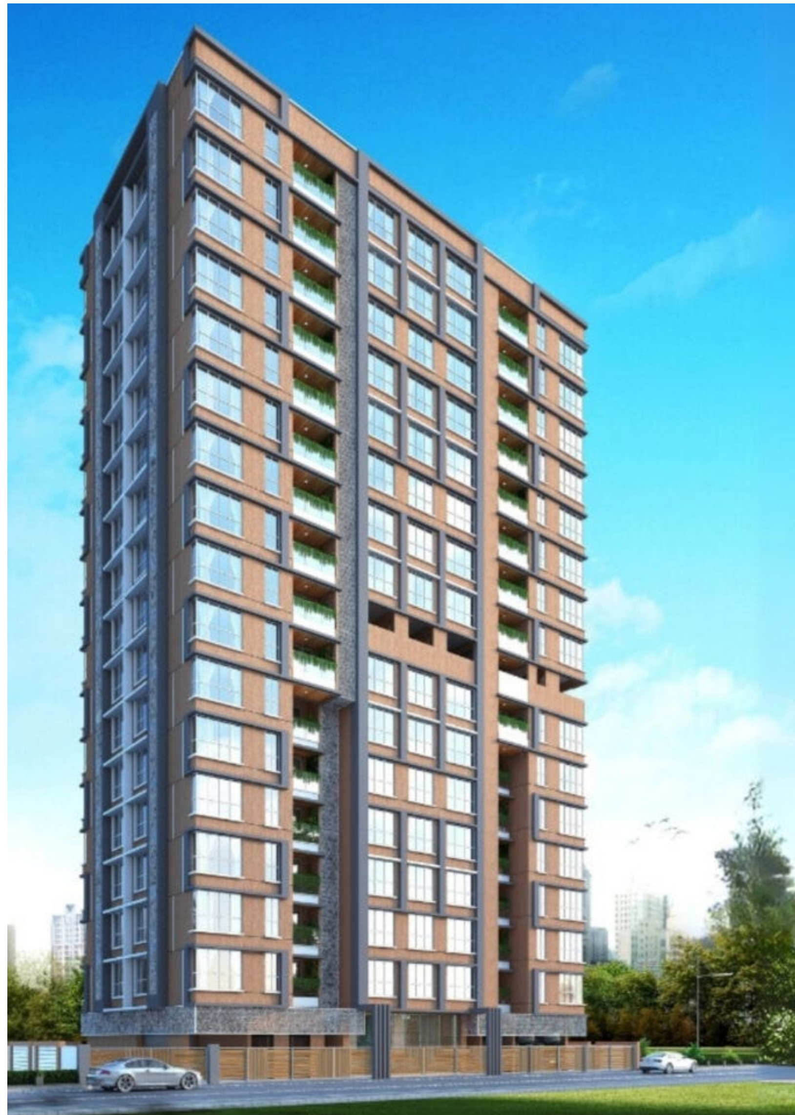
Ghatkopar Aryana [ Under Construction ]
